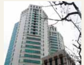
Shanghai Liaison Office (Shanghai, China)
