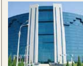
Uzbekistan Office (Tashkent, Uzbekistan)
