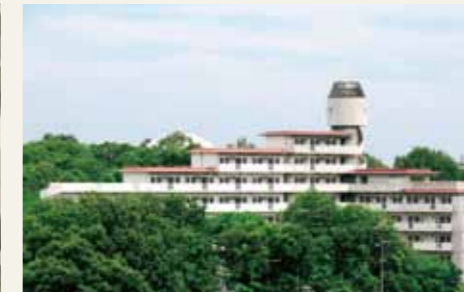
International Residence HIGASHIYAMA
