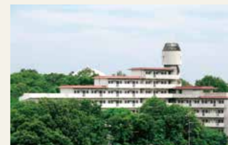
International Residence HIGASHIYAMA
