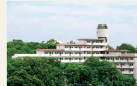
International Residence HIGASHIYAMA
