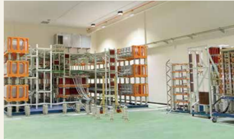
Figure 3 Lightning Strike Test Facility
